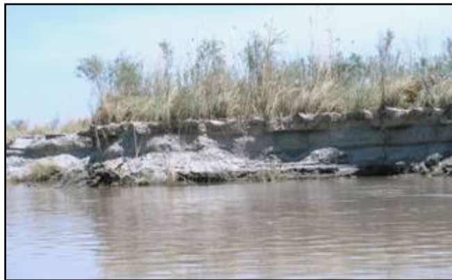
Image 2: River bank erosion
